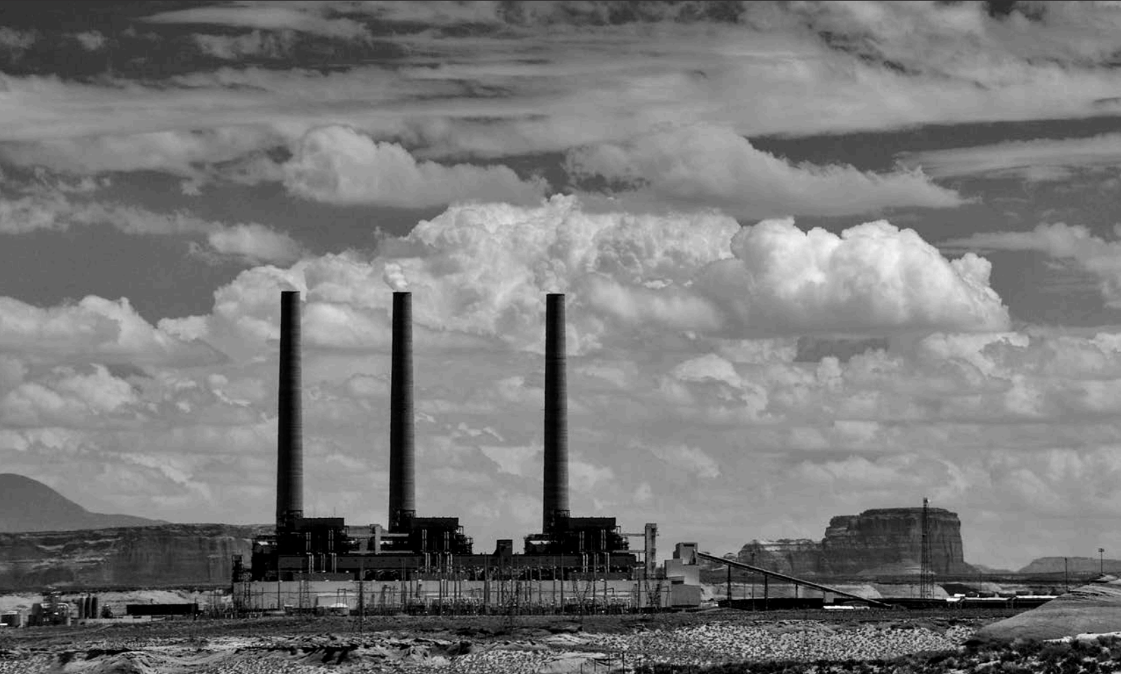
COAL POWER PLANT
