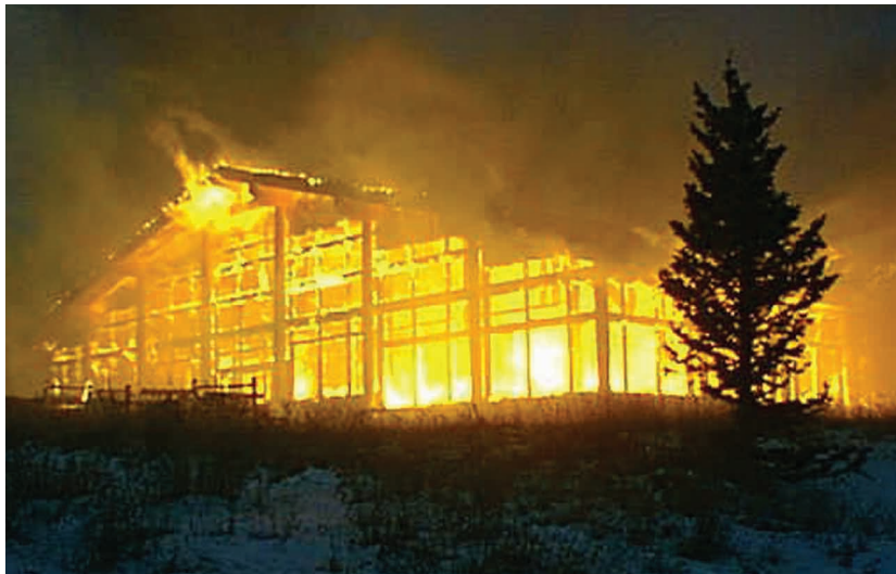
Ecoterrorists burned down the Two Elks Restaurant in Vail, Colo. in October of 1998; this was one of seven fires.
