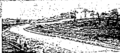
The first highway built exclusively for automobiles was this 45-mile, private toll road—the Long Island Motor Parkway.
