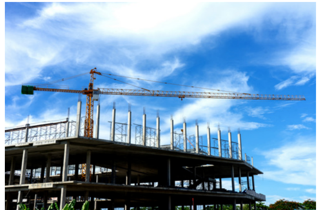
Commercial building site with crane. Source: Adobestock.
