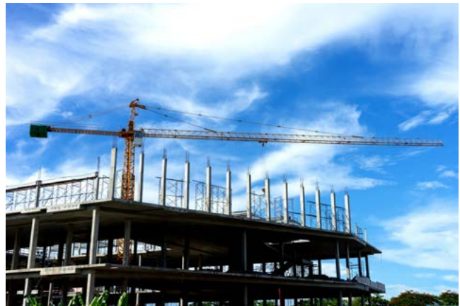
Commercial building site with crane. Source: Adobestock.
